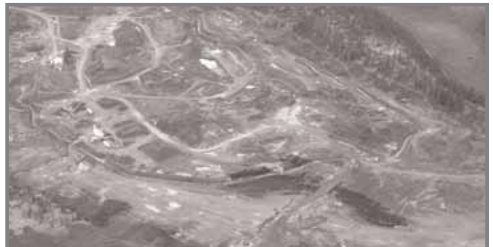
EPA is now enforcing wetlands and water quality violations at this Anchor Point gravel pit in response to Keeper's efforts. Wetlands filling violations visible at bottom.
