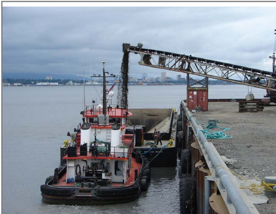
Loading barge with gravel at Port MacKenzie. Note closeness of Anchorage in background. Similar loading facilities in Seward are facing lawsuits from environmental organizations and public health advocates over Clean Water Act violations. What will prevent Port MacKenzie from facing similar costly litigation?
