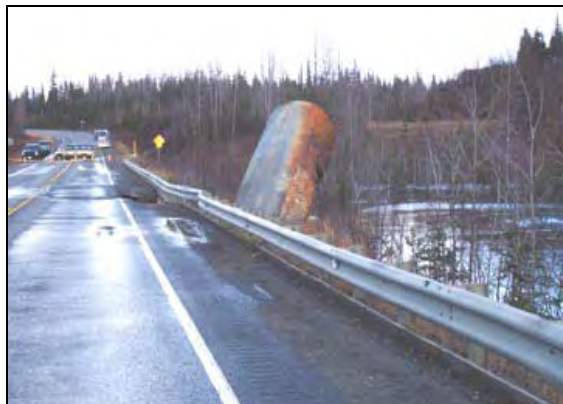
Culvert damage at Stariski Creek on the Sterling Highway, Oct. 2002. (Photo courtesy of J. Clutts)
