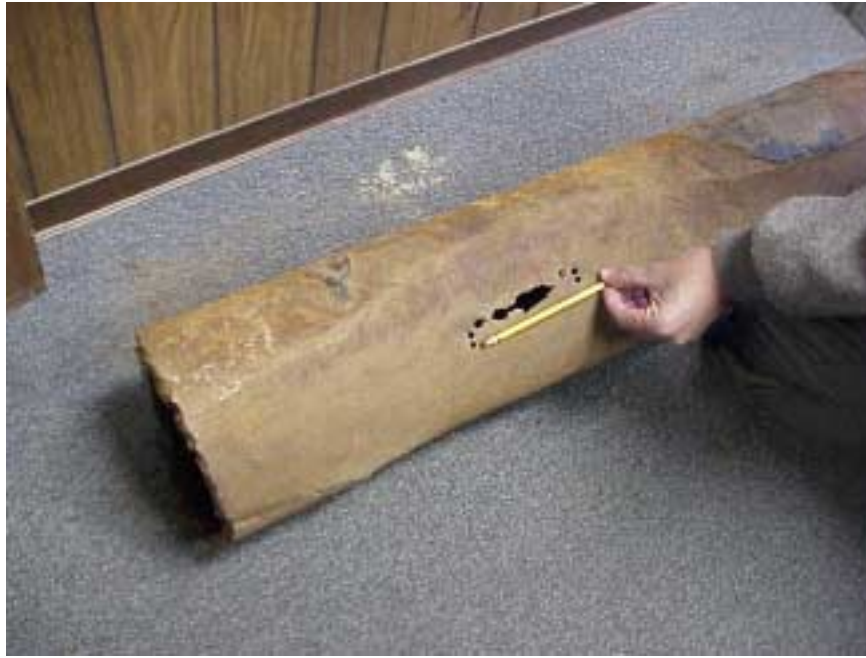
Figure 4. Photo of the Unocal 8” offshore oil pipeline which released 400-500 gallons of crude oil directly into Cook Inlet on October 23, 1999. The pencil shows the approximate length of the pipeline failure area. Photo source: Gary Folley, Alaska Department of Environmental Conservation (Soldotna office).
